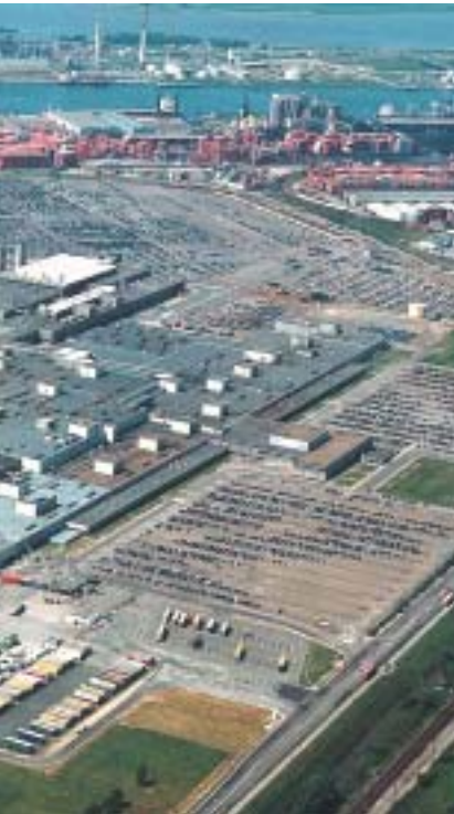
Above: This year a €340 million ($400 million) investment at Volvo's Ghent site has seen capacity rise to 270,000
